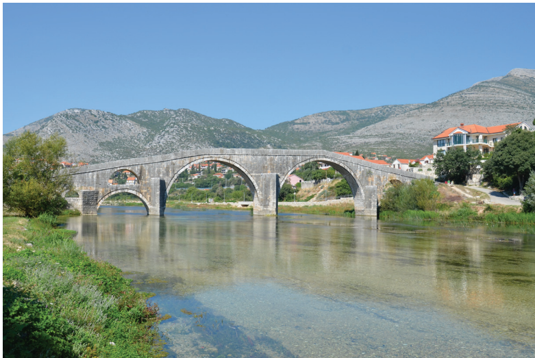
Arslanagica Bridge in Trebinje
